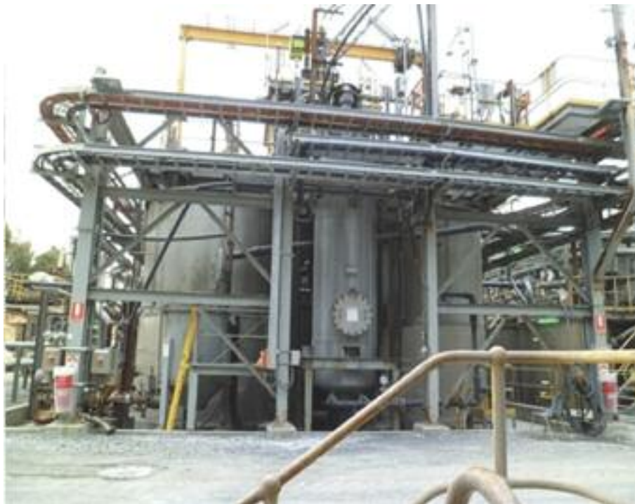
The Fosterville HiTeCC facility
